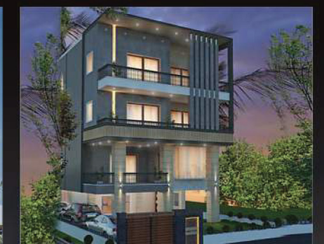
Mosaic House, Vaishali Nagar
